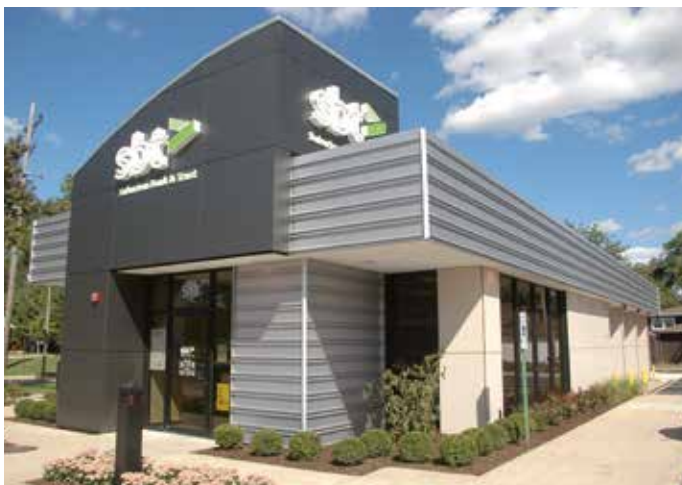
North Suburban Bank and Trust, Elmhurst, Illinois (USA)
